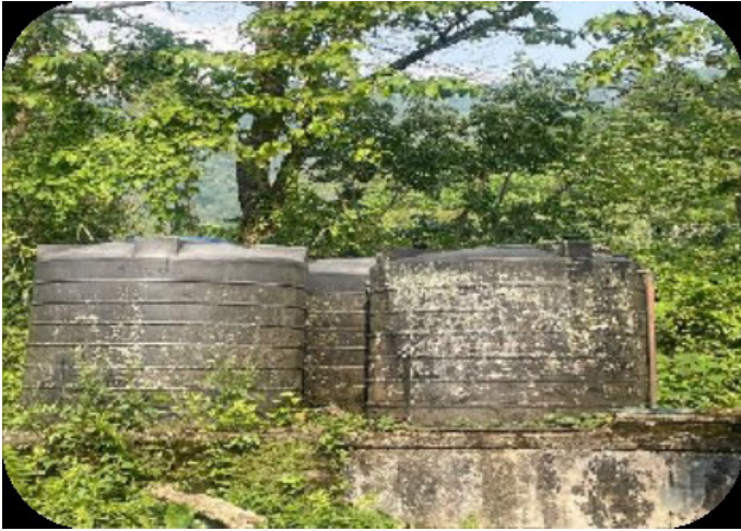
Water Tanks inside College
